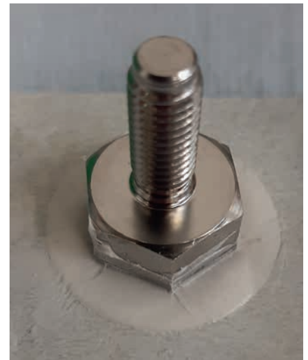
Repaired opening of PFP-coating
